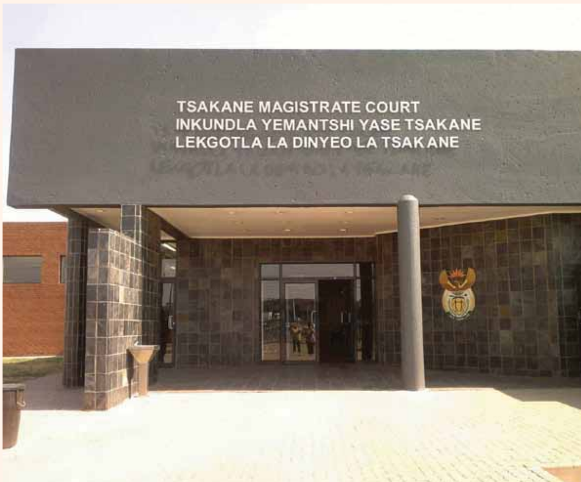
The Tsakane Magistrate Court in Gauteng was completed during 2011/12 to improve access to justice to the nearby community.
