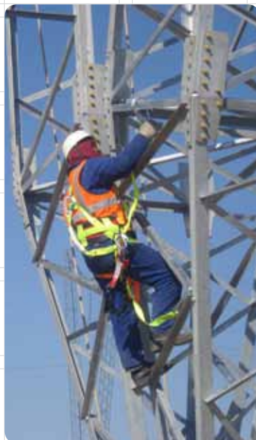
Employee and contractor safety remains a major concern
