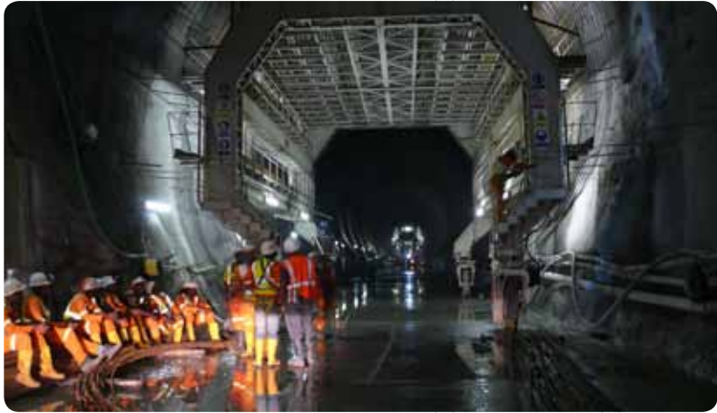
The Ingula pumped storage scheme near Ladysmith is built mainly underground
