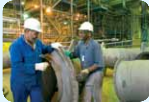
Restoration work at Komati power station
