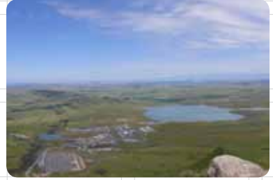
The Braamhoek dam is complete at the new Ingula pumped storage scheme
