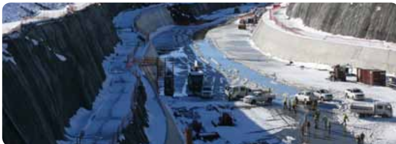
Snow covers the intake canal of the Ingula pumped storage scheme under construction near Ladysmith
