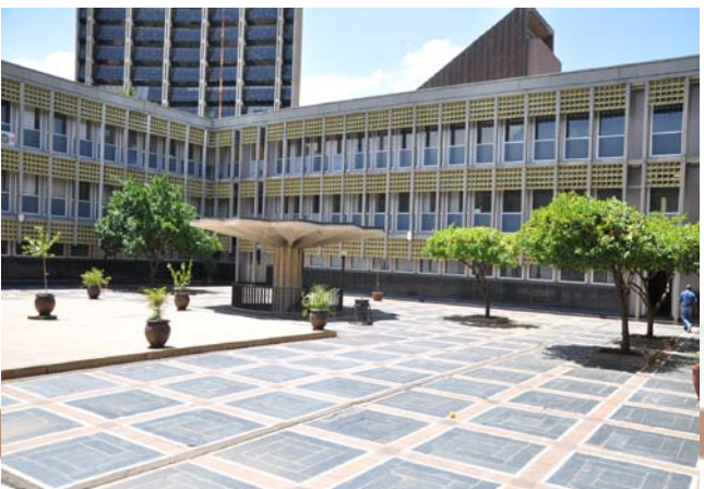
NIHE MAIN BUILDING
