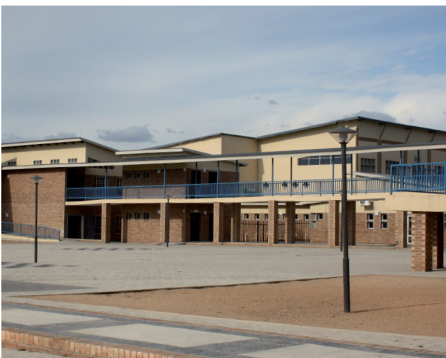
Completed Kamhlushwa Primary School project
