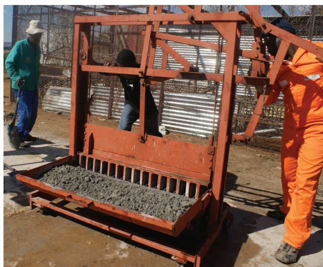
EPWP – Brick laying project
