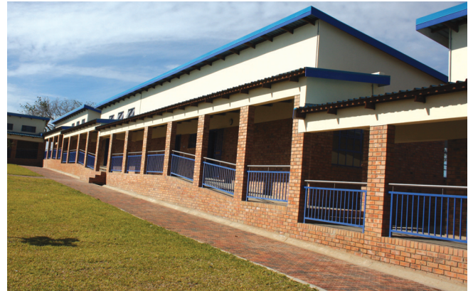
Kamhlushwa Primary School upgrade
