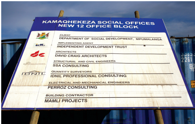
Construction of Kamaqhekeza social office
