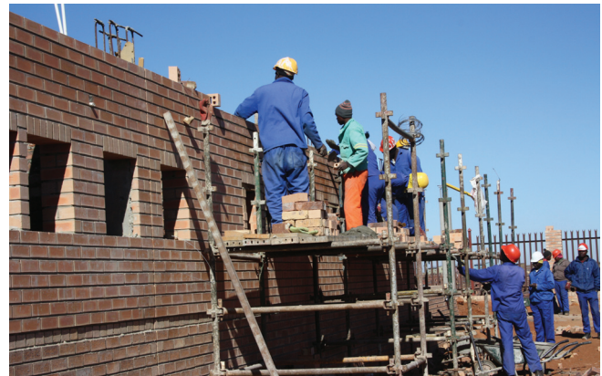
Construction of Kamaqhekeza social office
