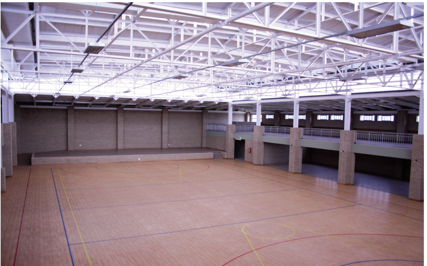
Sports centre at Cofimvaba Senior Secondary School
