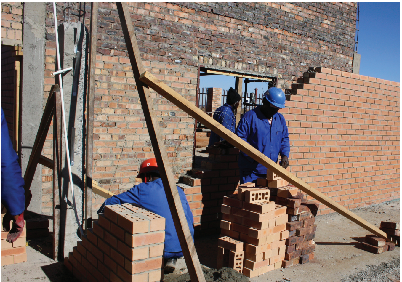
Construction of Kamaqhekeza social office
