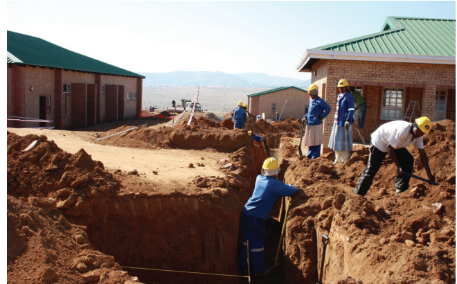
Photo Primary School in Glen Cowie village
