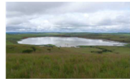
Ingula - Bramhoek dam
