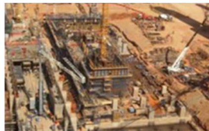
Kusile - Unit 1 Turbine Pedestal
