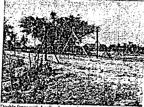
Double fence with 4 rolls of razor wire
