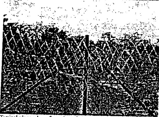
Typical place where fence is scaled at upright
