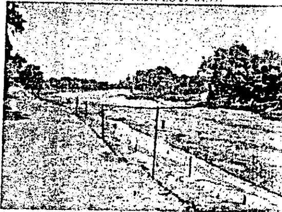
Single fence right at river bed
