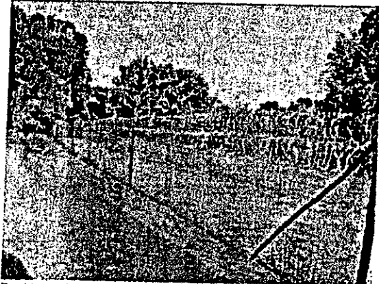
Double steel square wire fence with 4 rolls of razor wire
