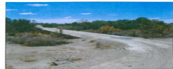
Bridge on access road to Eksteenskull.
