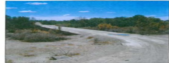
Bridge on access road to Eksteenskull.
