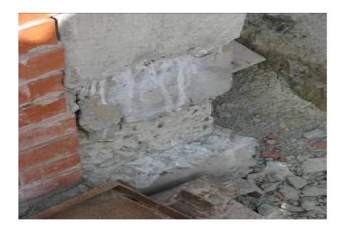
Photograph below depicts example of sub-standard work, e.g. support beams that have structurally been weakened, and poor brickwork.
