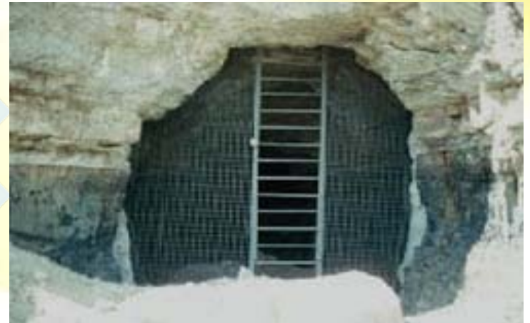
Bat grate installed on an abandoned mine in a conservation area in the USA
