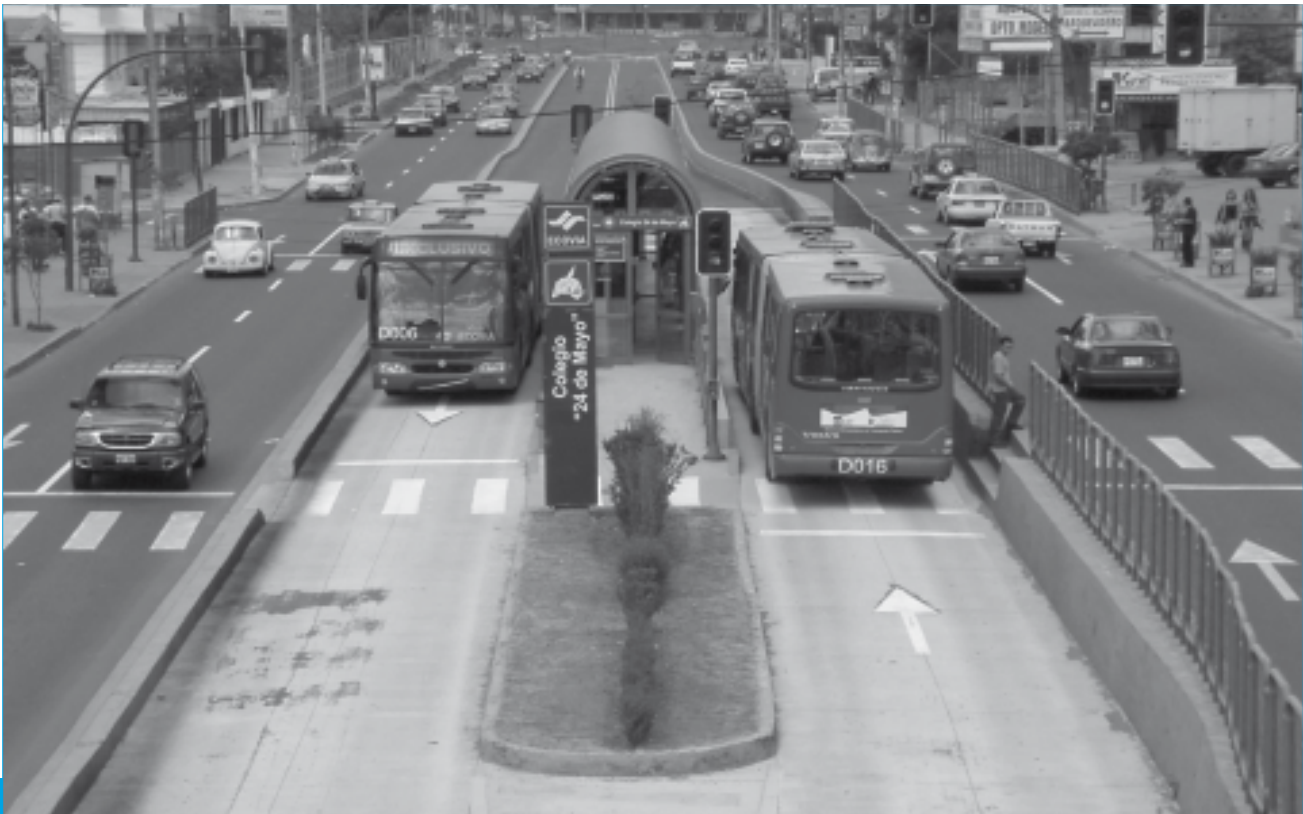
Figure 14: Transmilenio system showing median lane and station
