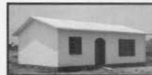
House constructed from gypsum panels
