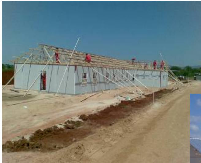
Mid April: Residence 1 at roof height
