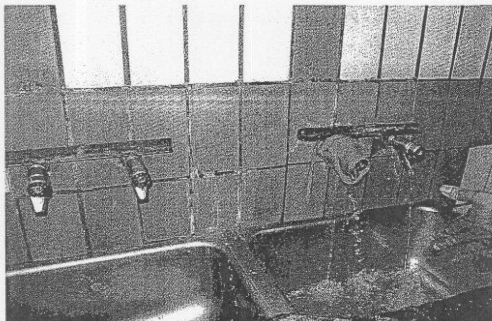
Copious amounts of water were constantly pouring from the taps and down walls.
