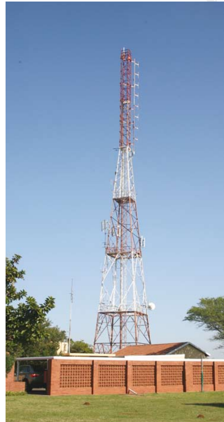
Transmitter Site, Durban Regional Office
