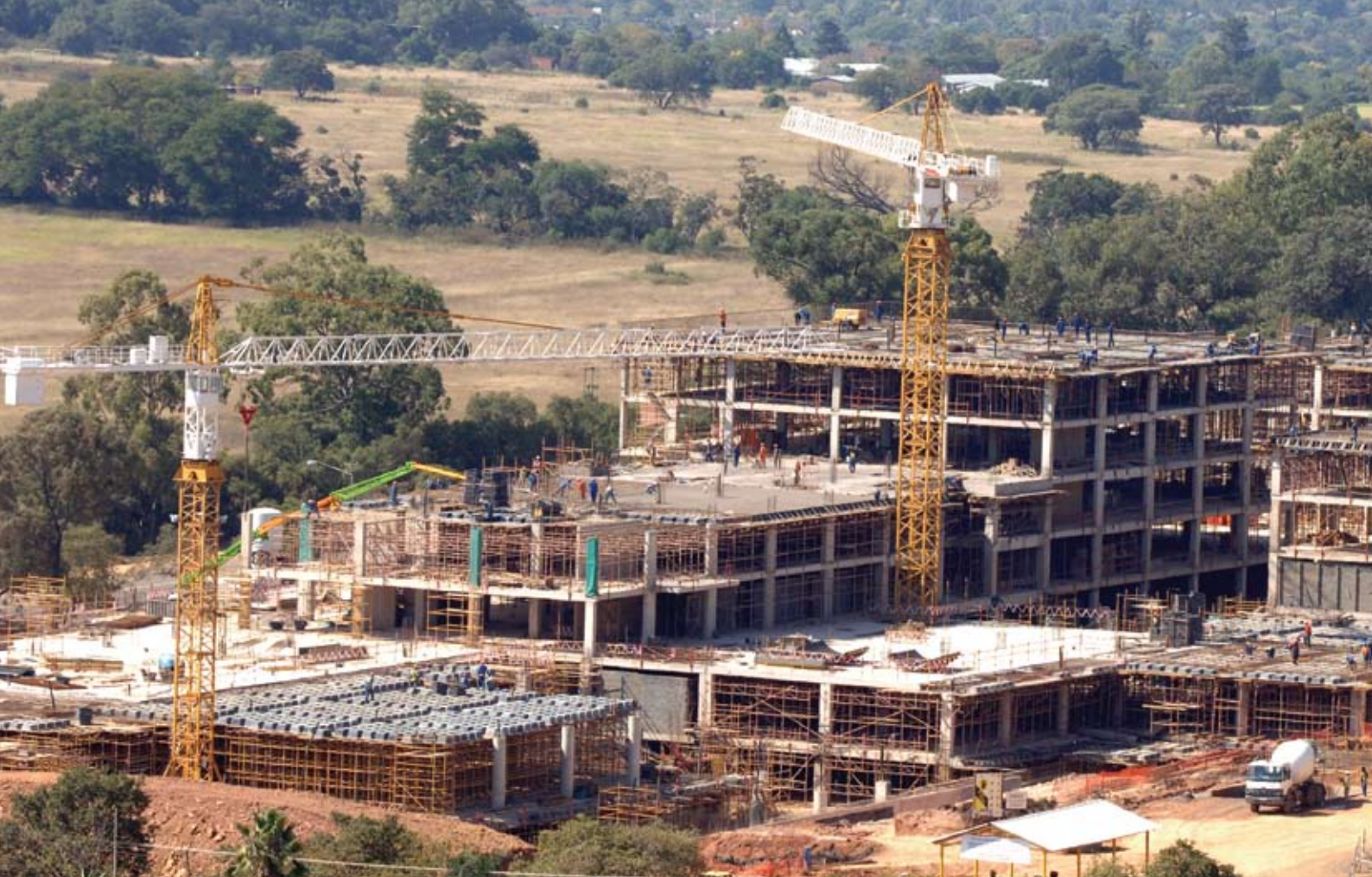
The new DFA Head Office under construction, Pretoria
