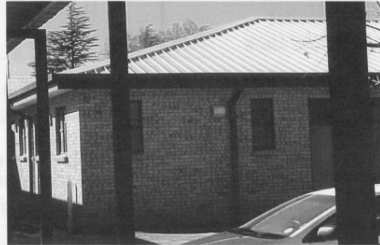
Delmas Maternity Ward at completion stage in June 2008
