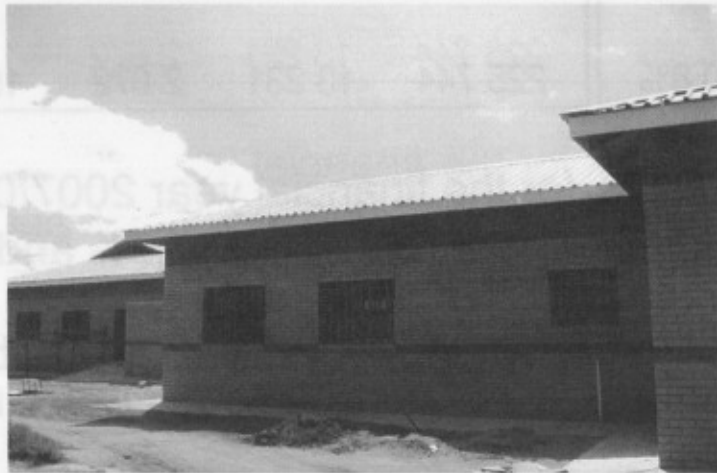
Ermelo Psychiatric ward at completion stage
