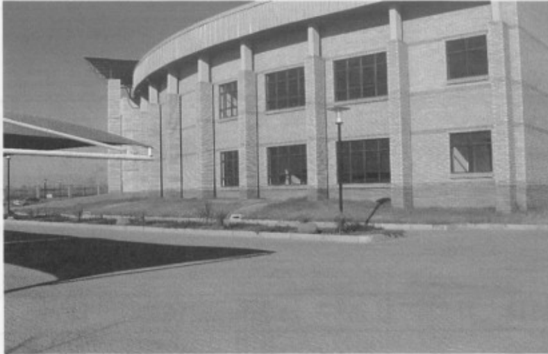
Middelburg Pharmaceutical Depot at completion in May 08
