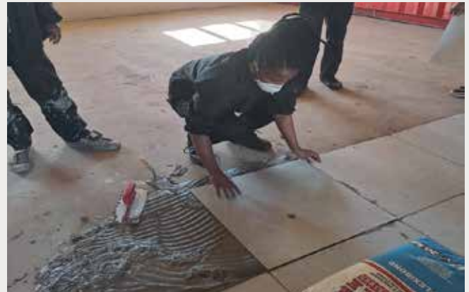
Dondotha Community Centre, in Dondotha, King Cetshwayo District.
