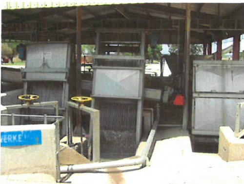
Figure 1 & 2 – Mechanical Screens
