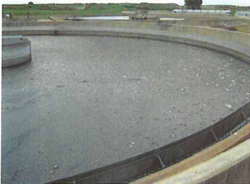
Figure 7 & 8 – Secondary Clarifiers
