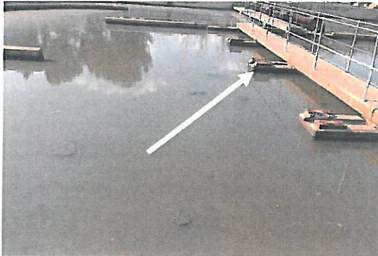
Fig9: Aerator removed
