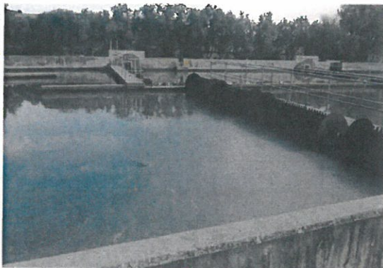
Fig4: Aerator not functional
