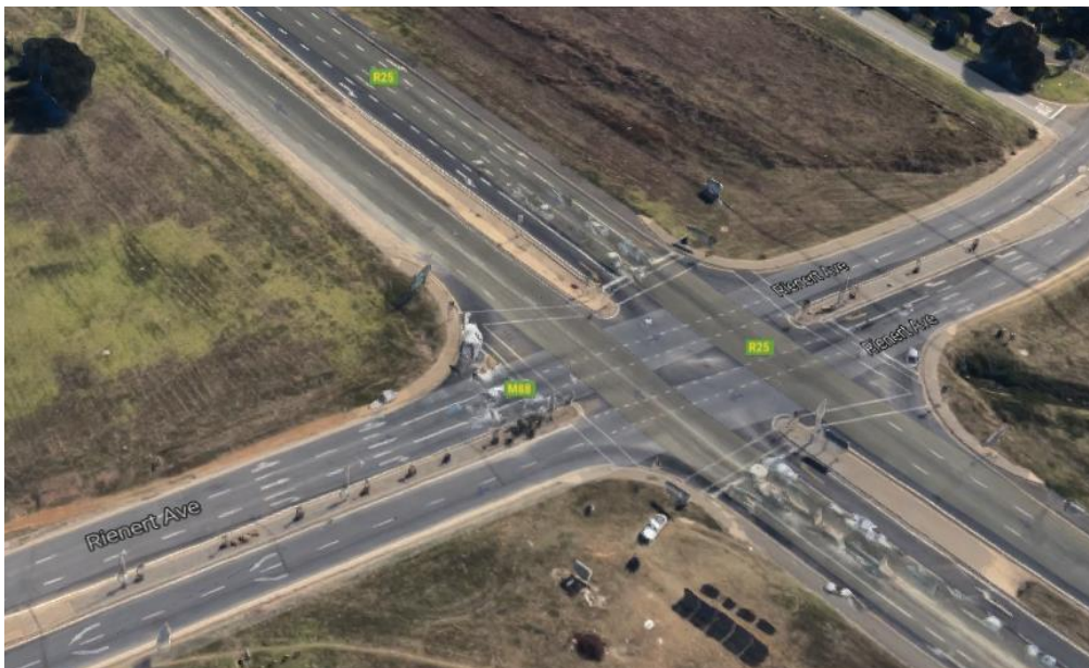
Figure 4-10: Intersection between M88 ( Rienert Avenue) and R25 ( Modderfontein Road)
