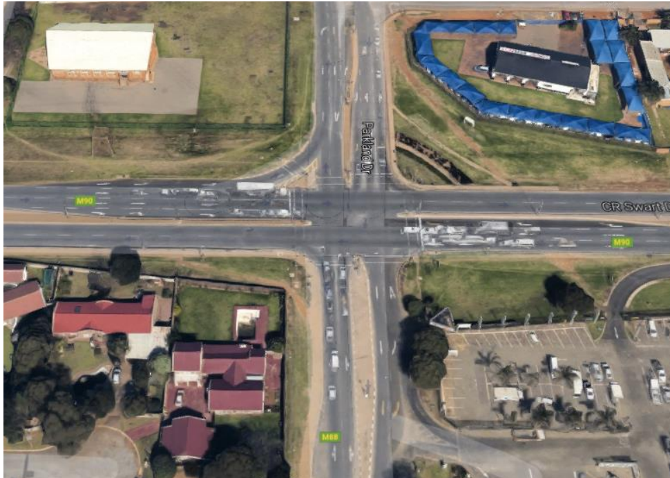
Figure 4-11: Intersection between M88 (to the north) and M90 (to the east)
