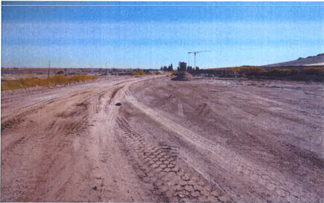
Figure 9: Cleanup completed around Kareerand TSF (outside containment area) - August 2018
