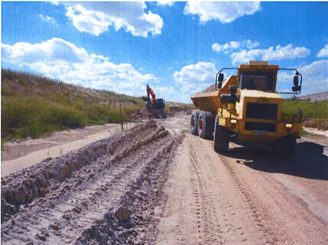
Figure 4: Clean-up in progress around Kareerand TSF (inside containment area)
