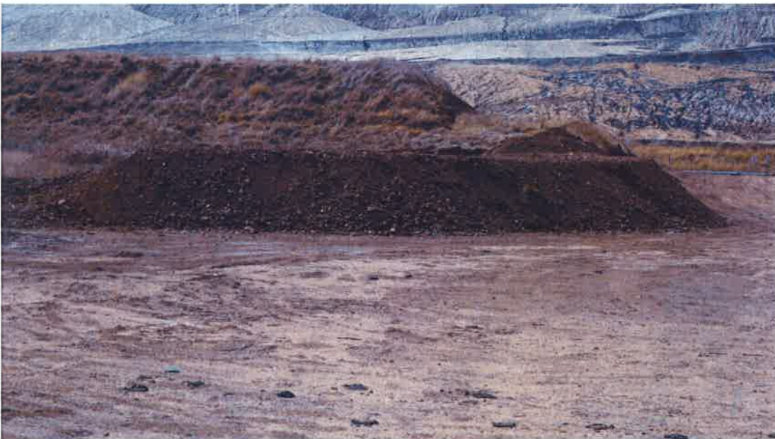
Figure 16: Clean storm water diversion culvert at entrance to Kareerand TSF
