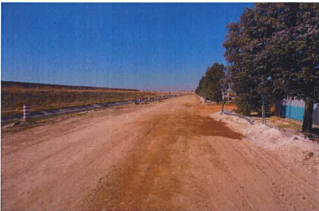
Figure 6: Cleanup completed around Kareerand TSF (inside containment area) - September 2017
