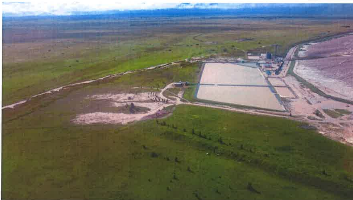
Figure 2: Spillage towards the Vaal River (21 Feb 2017)
