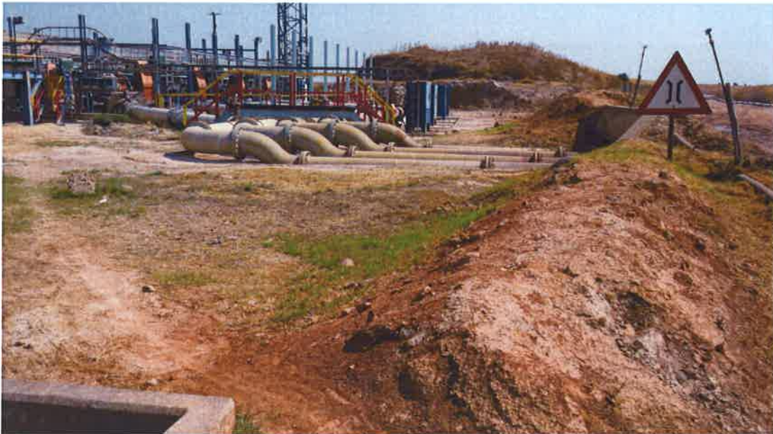
Figure 14: Rolled edge constructed to protect pump station and office
