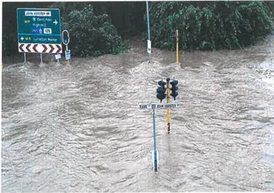
Figure 15: Poor drainage system
