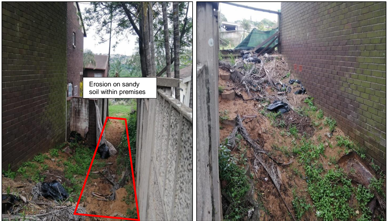
Figure 4-7: Corrosion path downhill along retainers
