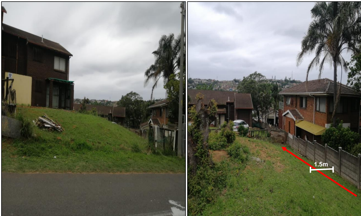
Figure 4-4: Slope Running Perpendicular to Affected Private Property Precast Concrete Slab Fencing
