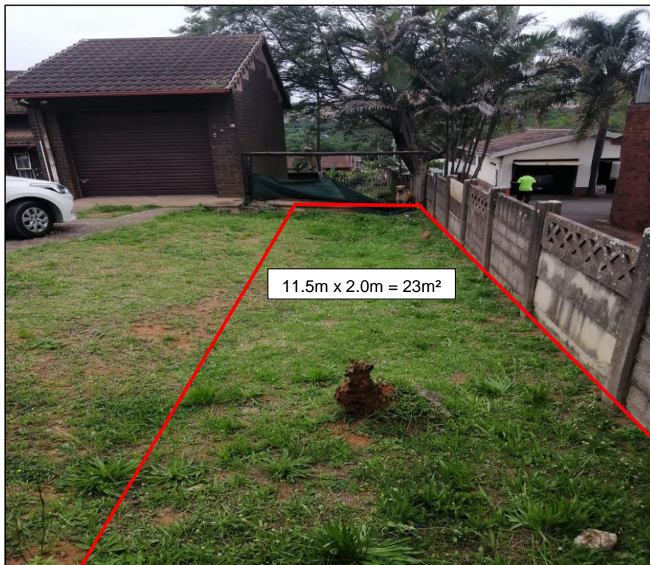
Figure 4-5: Channelling Point against Private Boundary Fence from 1 and 2 Periwinkle into Back Yard at 2 Periwinkle
