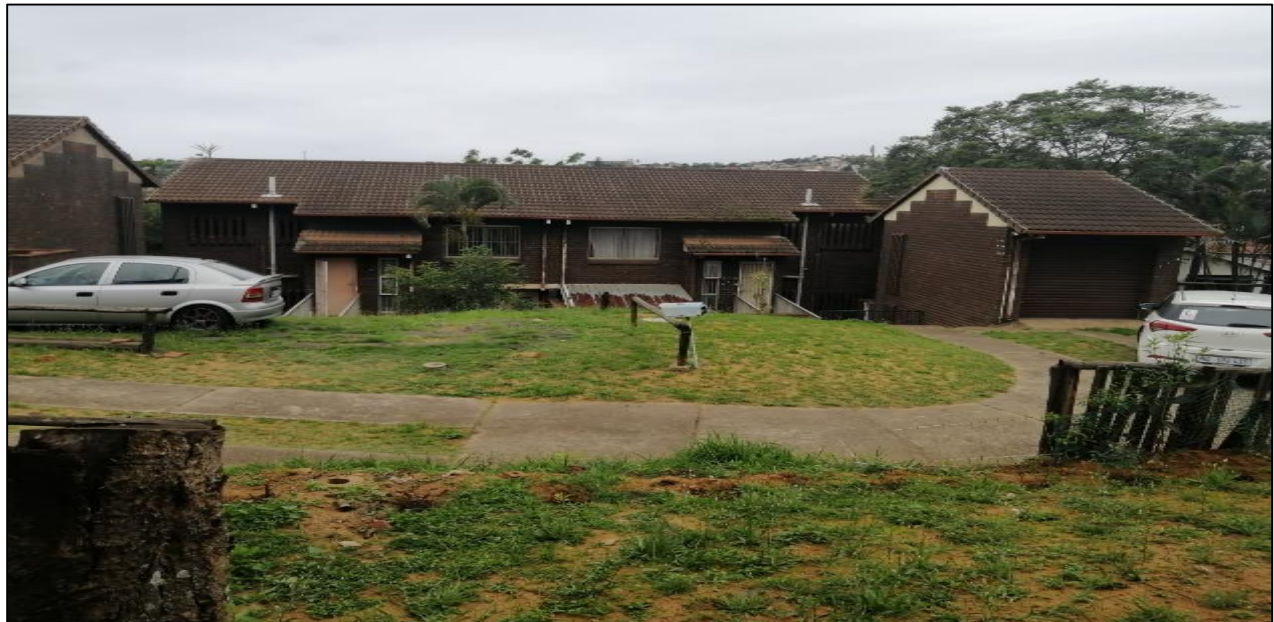
Figure 3-4: Entrance Level to Two storey Dwelling on the Top Level
