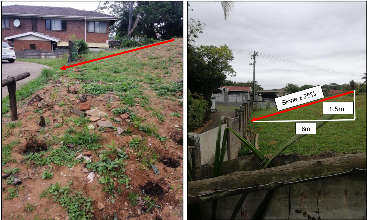
Figure 4-3: Slope Running Parallel to Affected Private Property Precast Concrete Slab Fencing
