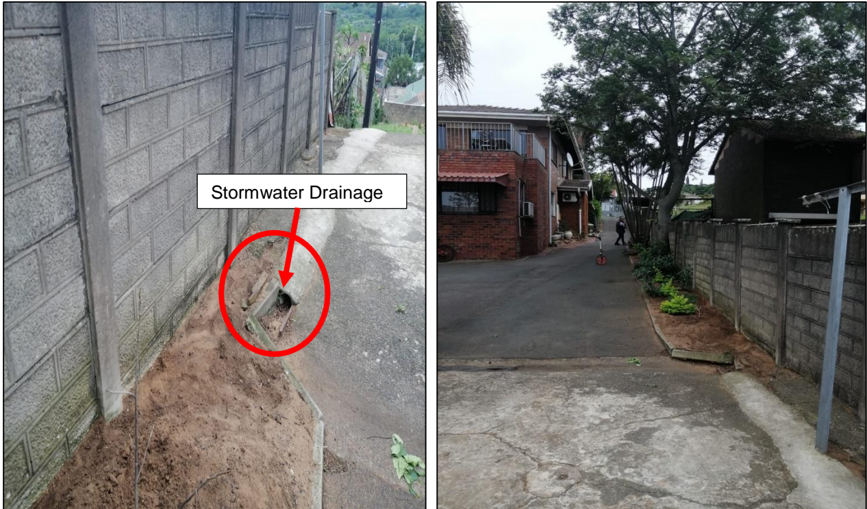
Figure 3-2: Private Dwelling - Site drainage, Surfacing and Precast Concrete Slab Fence
