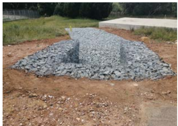
Area after installation of the Gabion and Reno mattress.
