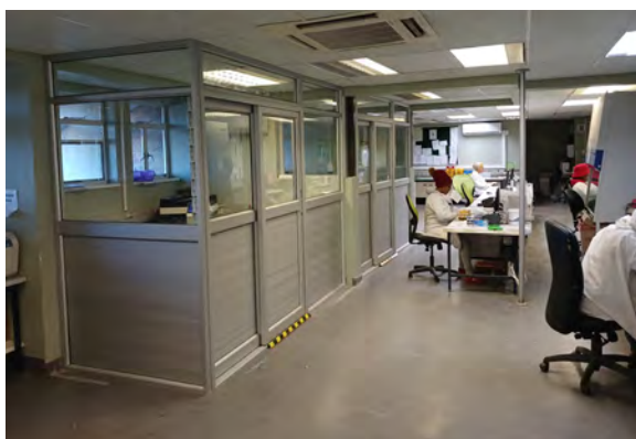
Figure 10: Renovations at the Kimberly Core Laboratory staining laboratory.
