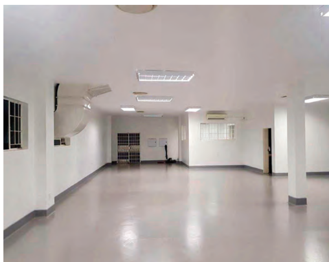
Taung phase 1: Flooring and painting
