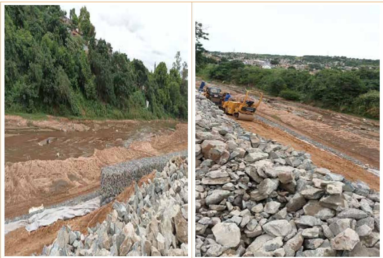
Figure 42: Peace palm close Phoenix Storm water project (eThekwni, KZN)
