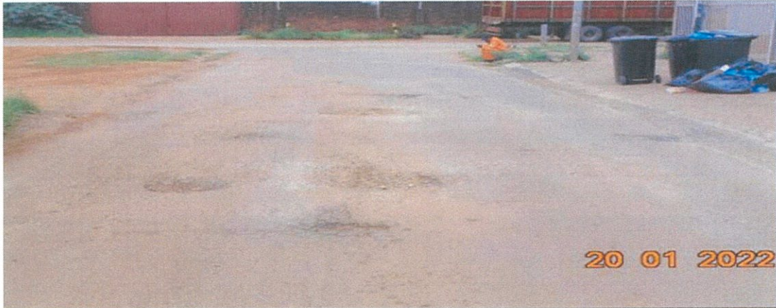
Figures 46: Eltivillas project before rehabilitation
