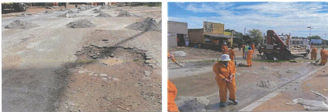
Figure 47: Malamulele section B and section C during rehabilitation
