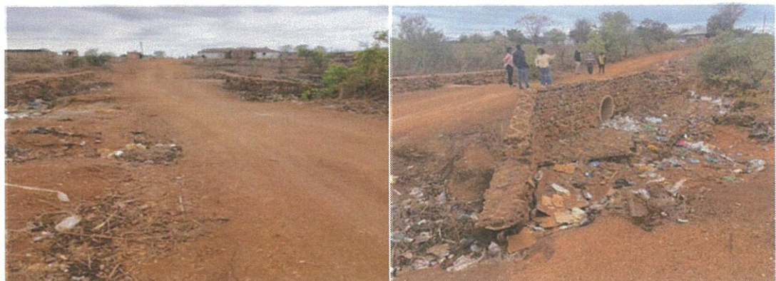
Figure 48: Makuleke culvert bridge project, in Collins Chabane Local Municipality
