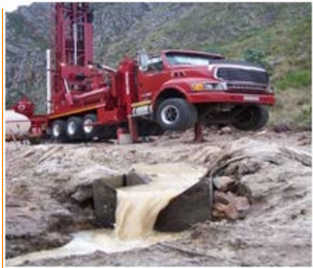
Drilling in progress
