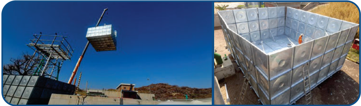
Installation of the Olifantspoort Scheme Service tank
