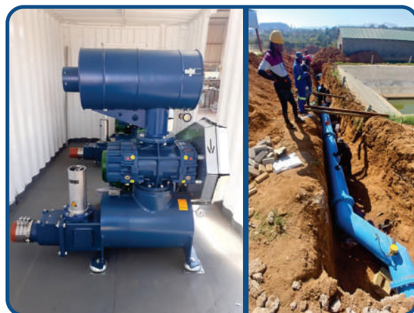
Burgersfort WWTW upgrade and refurbishment project
