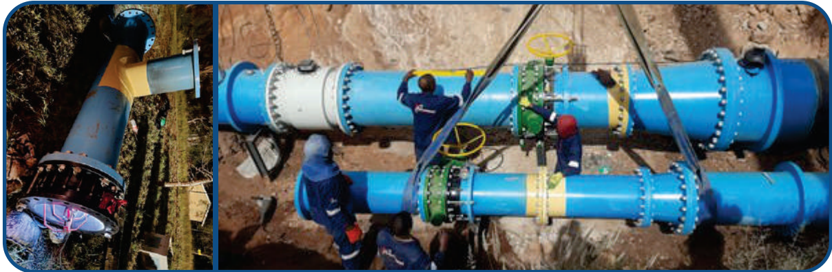
PMC valves replacement project at the Phalaborwa Scheme
