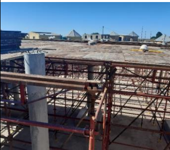
1 ML Reservoir Upper Ngqwara : Roof Shuttering
