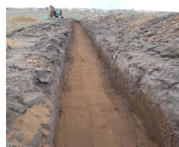
Pipeline: Pipeline trench backfilling.
