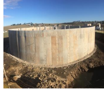
1ML Reservoir Upper Ngqwara: Reservoir Wall
