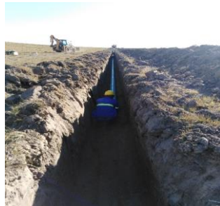
Pipeline: Laying of 355mm pipe class 16
