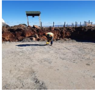
500 KL Reservoir Viedgesville : Testing of stabilized G5 layer.
