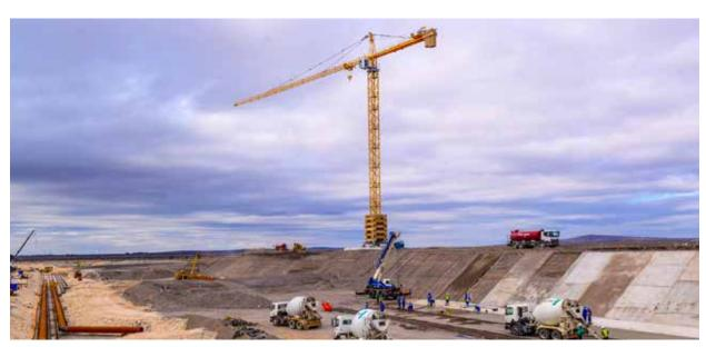
Construction of eight crude oil storage tanks, with a capacity of 1.1 million barrels each, has begun in the Port of Saldanha, Western Cape.
