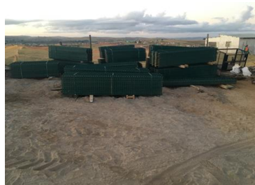
Material on site- Reservoir Wall Shutters
