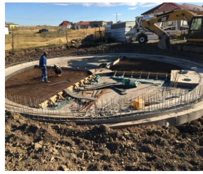
500 KL Reservoir Zwelitsha- Floor Quadrants steel fixing.
