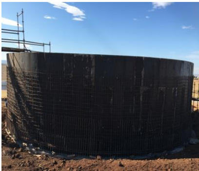
1ML Reservoir Mandlovini- Steel fixing and wall shuttering
