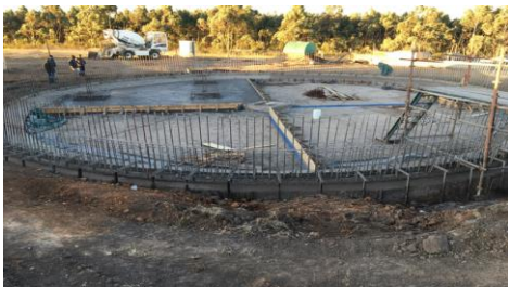
1ML Reservoir Cezu - Floor Quadrants steel fixing
