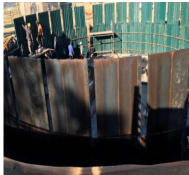
500 KL Reservoir Maqomeni- Steel fixing and wall shuttering.
