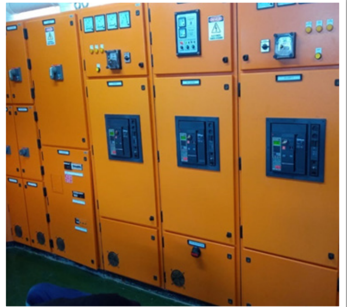
Bulk meter replaced and new electrical panel built
