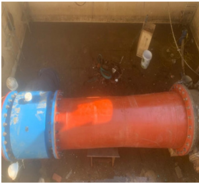
Bulk meter replaced and new electrical panel built
