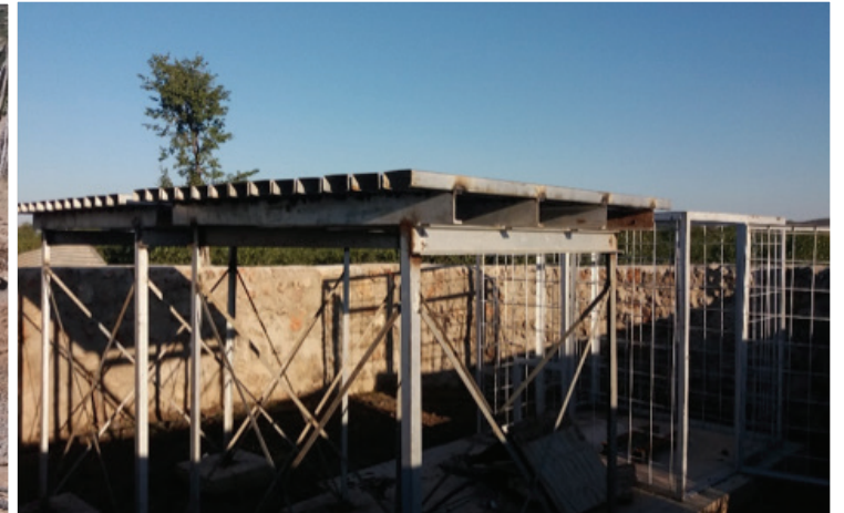
Tank stand protected by elephant wall
