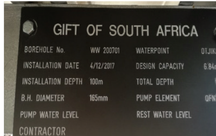
Name plate: Branding with borehole details
