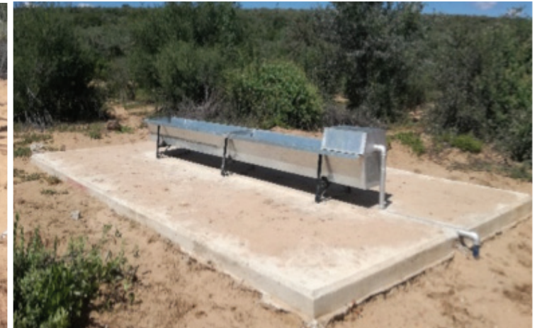
Drinking trough and on concrete apron
