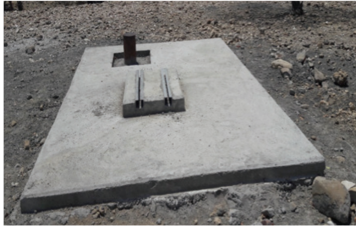
Borehole concrete and engine stand
