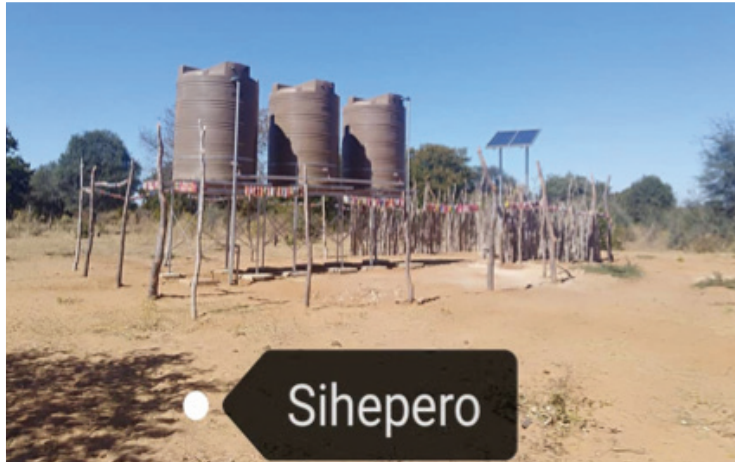
Completed borehole installation
