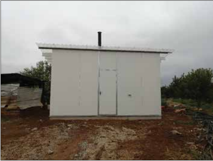
Front of the solar drying and storage unit constructed in Mukula.
