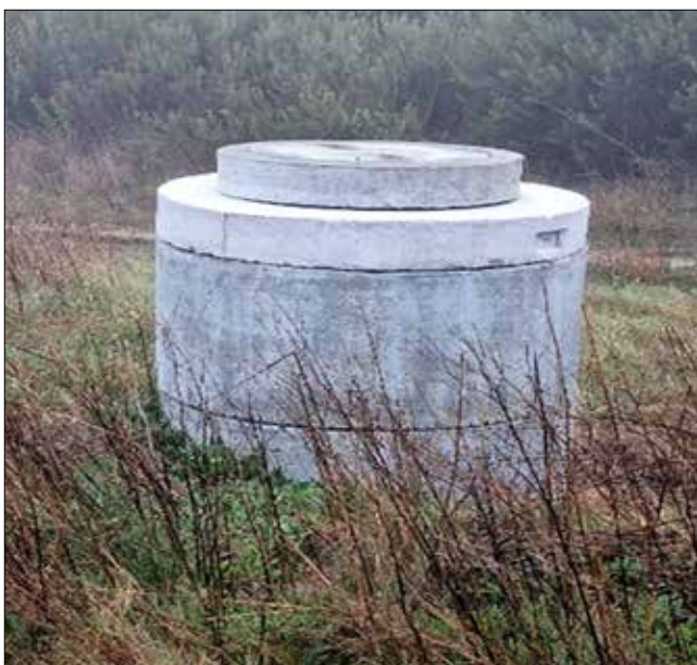
Second borehole that has been enclosed with concrete rings in order to protect it.
