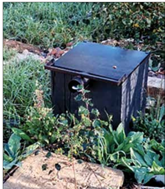
Borehole safely secured and tamper free.
