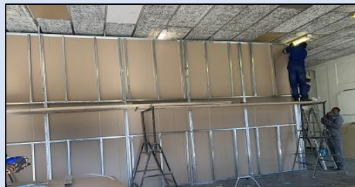
Hall preparation still in early stages
