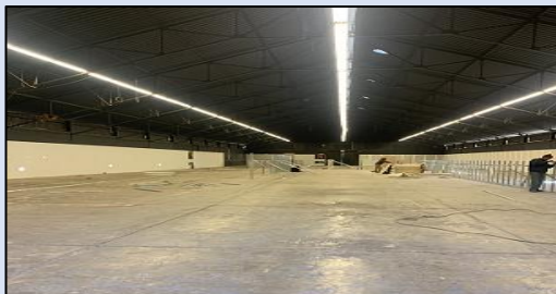
Drywall installation in progress
