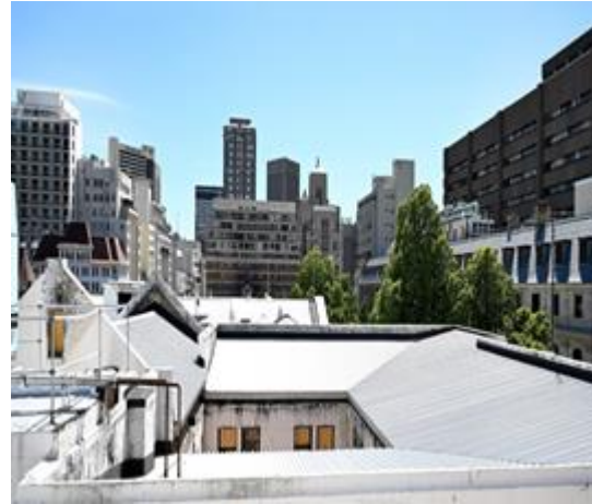
Temporary Roof Installed at OA
