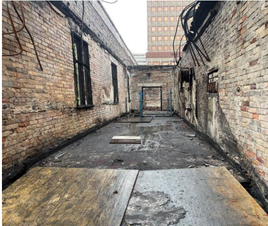
Rubble Removed from OA
