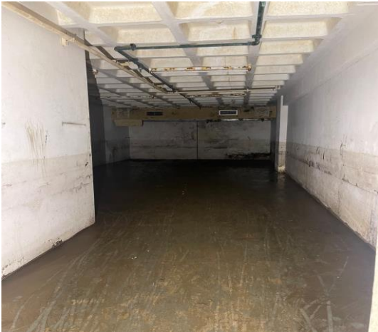
LB Storeroom Cleared
