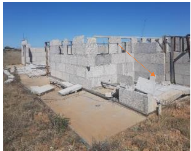
Figure 8: Collapsed wall
