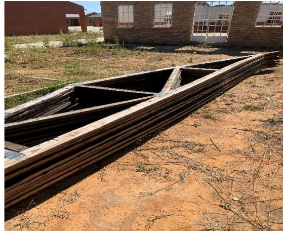
Figure 14: Weathered trusses
