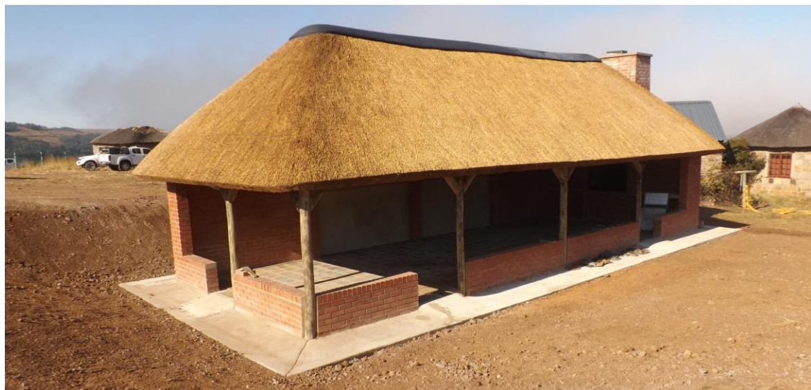
Constructed lapa in Madlangala
