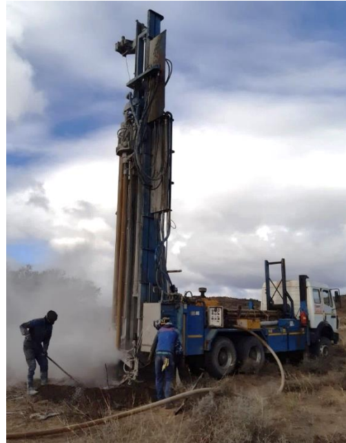
Drilling Borehole at Merweville
