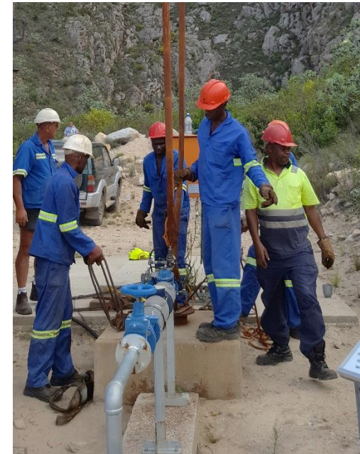
Inspection of existing boreholes
