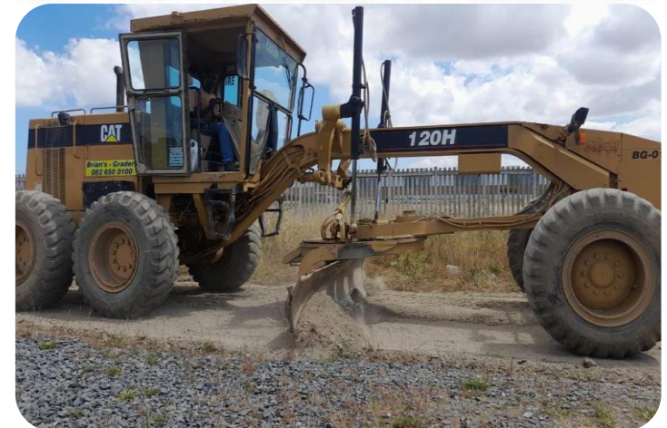
Grading Service Roads
