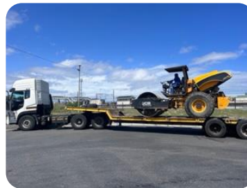
Some of the equipment used
