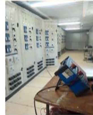
Ugesi Relays continues to perform pre-commissioning testing
