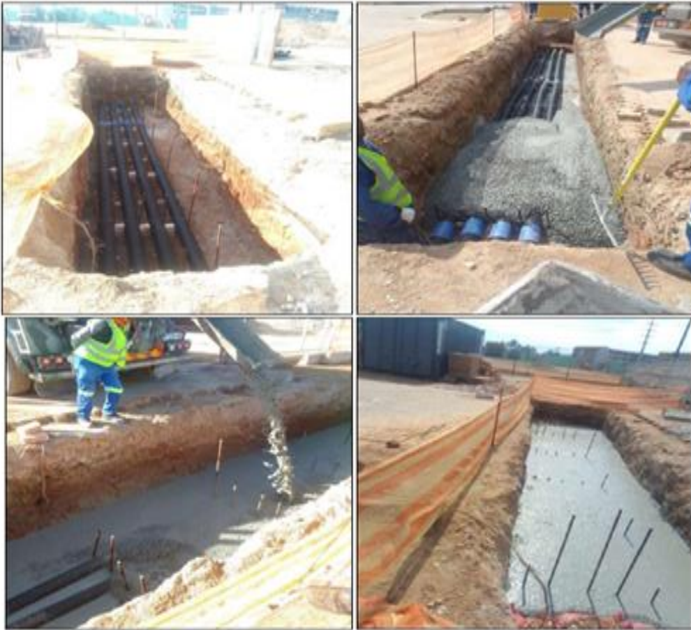
Installation of MV cable sleeves under substation road
