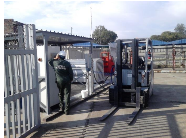
Fuel Cell Forklift refueling station
