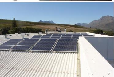
The ARC made investment in solar projects at Infruitec Campus. The post harvest cold rooms are fitted with 224 solar panels housed on the carport, generating 75kva and the Nietvoorbij cellar fitted with 16 solar panels which generates 25kva and provides power to the cold-rooms/freezers in the building.
