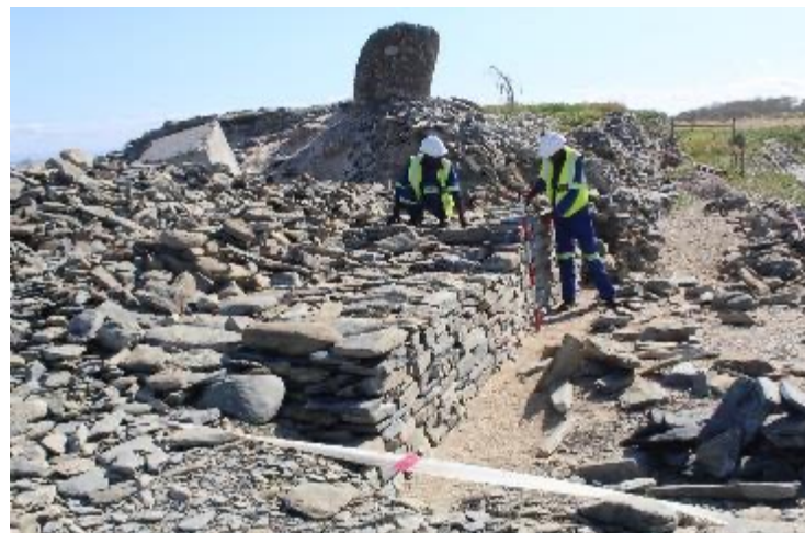
Figure 2: Wall restoration in progress
