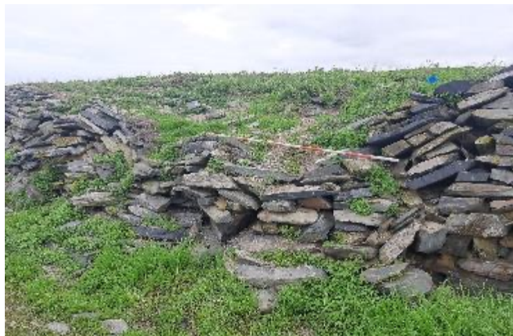
Figure 1: The left section of the wall before restoration
