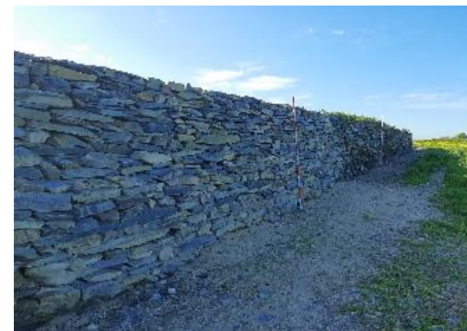
Figure 3: Front section of the wall restored
