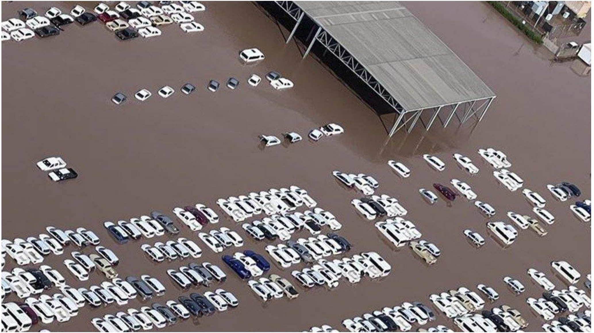
Toyota plant in KZN – damage caused by floods
