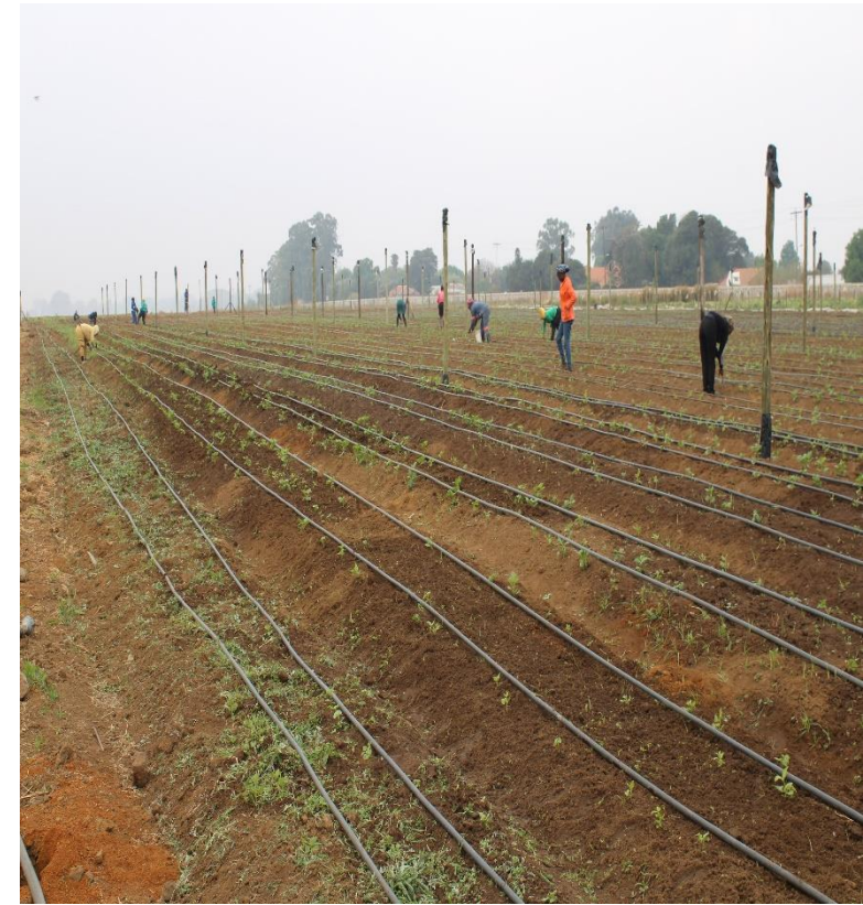
Laying of irrigation and constructing of shade cloths, in preparation of planting of spinach
