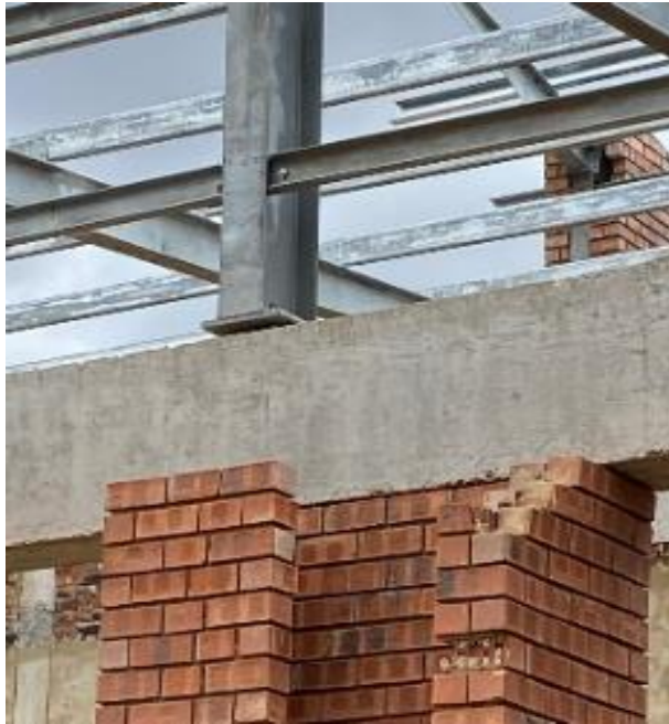
Mmabatho Nurses college (NW) - Brickwork incomplete and the steel column above the upstand beam not within the width of the beam and the construction of a staircase that is not in accordance with building regulation SANS10400-M, MM2.3. The step of the staircase is exceeding allowance of 200mm.
