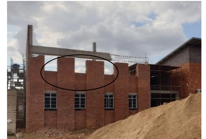
Mmabatho nurses college (NW) - Inadequate load bearing columns for the span of the concrete floor slab above.
