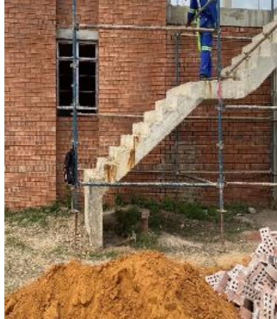
Mmabatho Nurses college (NW) - Brickwork incomplete and the steel column above the upstand beam not within the width of the beam and the construction of a staircase that is not in accordance with building regulation SANS10400-M, MM2.3. The step of the staircase is exceeding allowance of 200mm.
