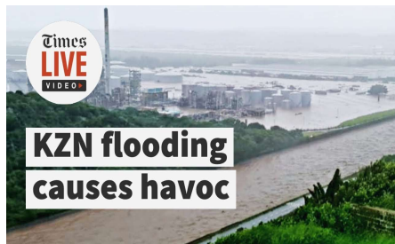
Damaged buildings due to KZN disaster floods)
