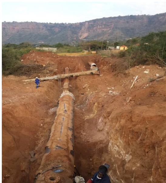
Site 3A Exposed
