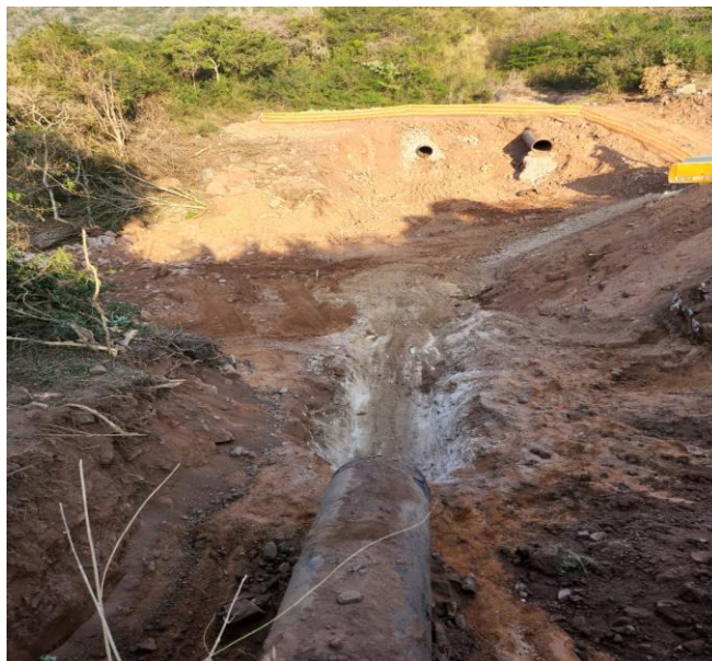
Site 3B Exposed
