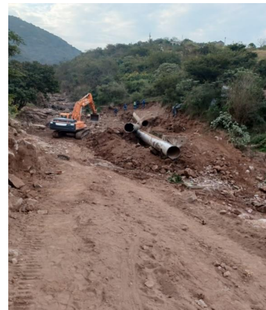
Site 4B Exposed
